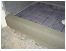
(5) Fill balance of curb with mud and screed top and sides.
