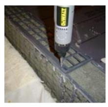
(4) Install top panel using the (8) 3/4" stainless, self tapping screws supplied. (Be sure the arrows on top panel are pointed to inside of the shower. Do not over tighten).
