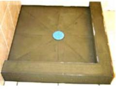
(6) Let curb dry over night and use a latex modified mortar to set tile. (Note: We recommend a roll-on waterproofing membrane to be added to the surface of the curb for additional protection prior to the installation of tile.)
