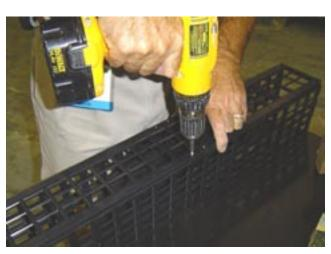
(2) Attach top panel to assembled side panels using the (8) 3/4" stainless self-tapping screws supplied. (Be sure the arrows on top panel are pointed to inside of the shower. Do not over tighten.)
