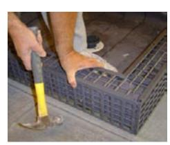
(4) Fit assembled curb over membrane wrapped 2x4s, attach with galvanized nails (not supplied) to the exterior only. (Caution: Do not nail to inside of curb, doing so will jeopardize the integrity of the liner!)
