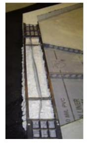
(3) Fill curb with mud just short of top. (We recommend a light weight wall mud for ease of workability.)
