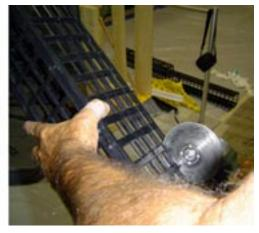
(1) Trim inside panel to allow for prepitch, using snips, hack saw or grinder.
