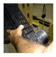
(3) Trim inside panel to allow for pre-pitch, using snips, hacksaw or grinder.
