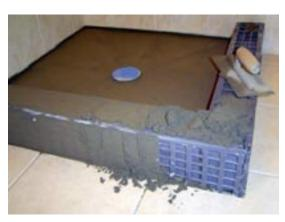
(5) Pack and fill side and top panels of attached curb with mud. <u>(We</u> recommend a lightweight wall mud for ease of workability.)
