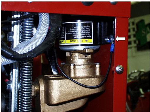
8. Attach other part of hose to inlet of water pump
